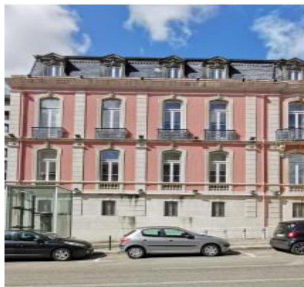
Fig. 7: East facade of the Mouzinho da Silveira Street mansion. Photograph courtesy of Hélder Carita.
