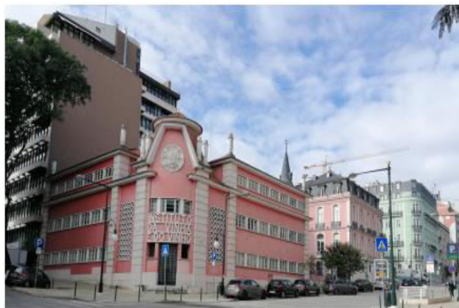
Fig. 6: Cassiano Branco, New building of the Wine and Vineyard Institute, 1943. Photograph by the author.
