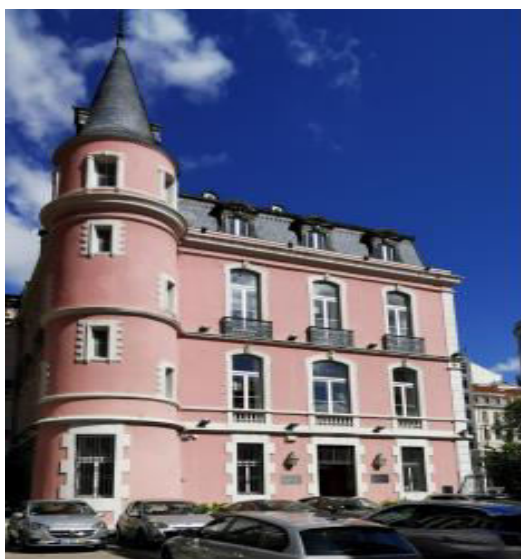
Fig. 8: South facade initially turned to the garden. Photograph courtesy of Helder Carita.
